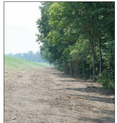
The result of the crew's clearing.
