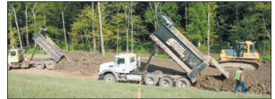
474L – Unloading borrow material.
