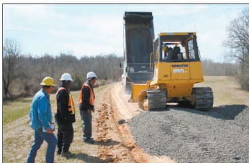
Dumping and spreading limestone.
