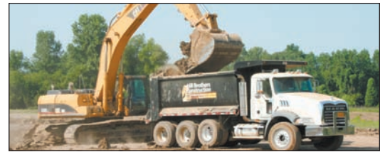
474L – Loading borrow material.
