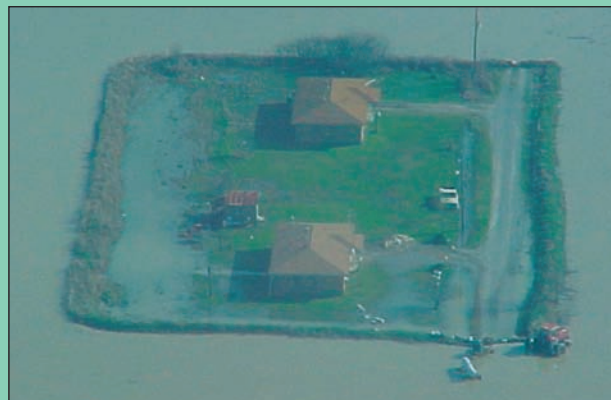
Flooding in the Darlove, MS area in December 2001.
