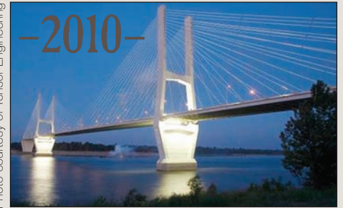
New completed Hwy 82 MS River Bridge.
